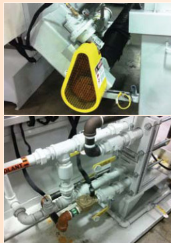
Plate and Frame Heat Exchanger used to control coolant temperature
